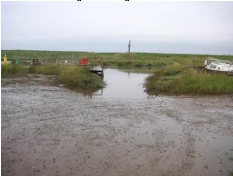
Existing slipway at point B, following high spring tide
